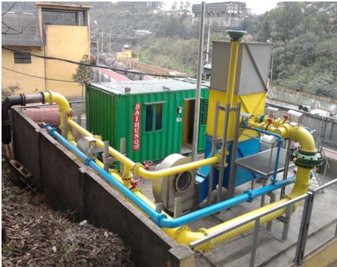
Gas Drainage Station, Khe Cham Coal Mine
