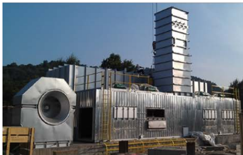
Duerping Mine (China)
