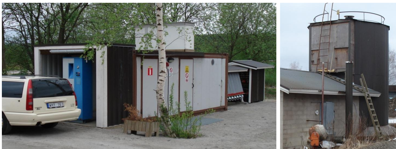
Figure 2.2. CBG filling unit, water scrubber based upgrading unit and high pressure gas storage (a) and biogas reactor (b) at Kalmari farm in Laukaa, Finland.
