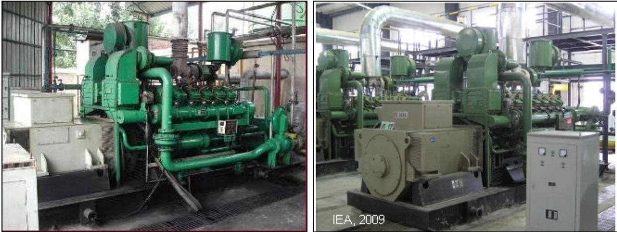
Figure 5-6: 500 kW Shengli Reciprocating Engine and Generator
