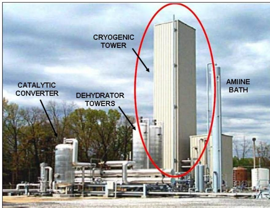
**Figure 5-7: Cryogenic Gas Processing Plant**
