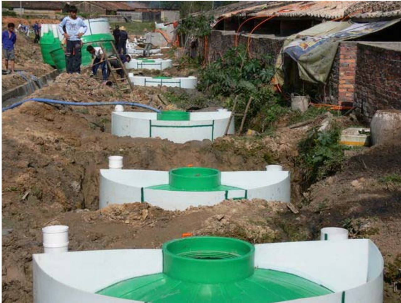
中国农村沼气建设 Village gas construction in China
