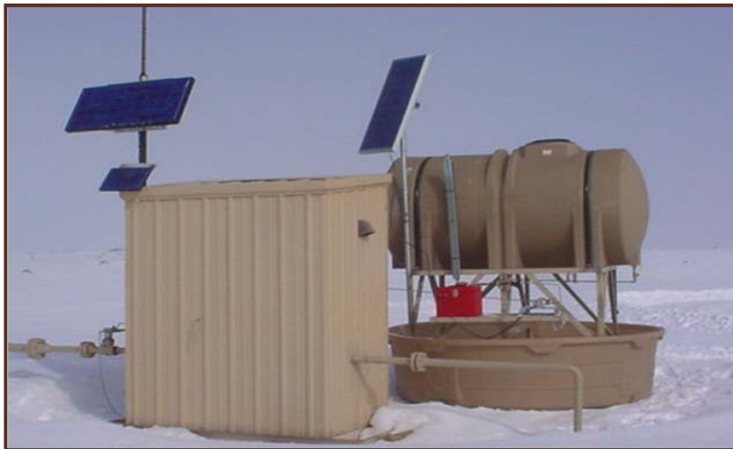
Source: Anadarko, Solar chemical pump
