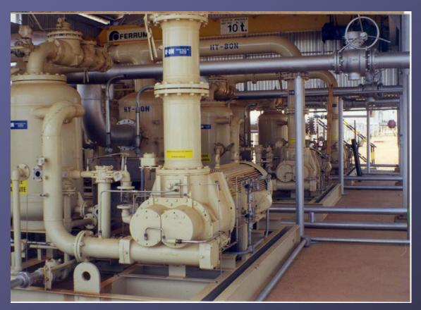
At this location, three of our compressor packages were set in tandem to move 15 MMSCFD of 2500-2600 BTU tank vapors.
