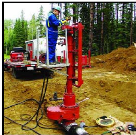
Certified Williamson Industries Technician performing a hot tap with a 760 Tapping Machine as part of a 12" Stopple application.
