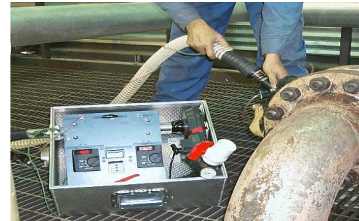
Oil and Gas Systems
