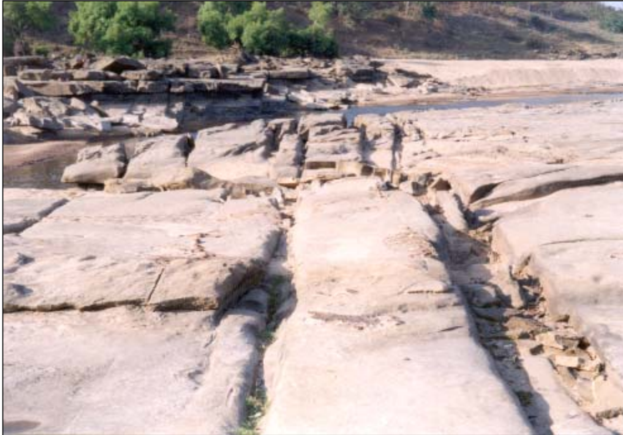
E-W major joint cut across by N-S joint, Kaser nala section
