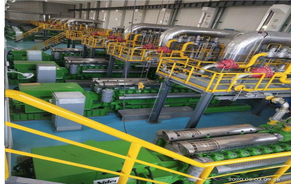
New CMM power project with total capacity of 30MW, using GE Jenbacher gas engines at Shihao Coal Mine of Chongqing City.
