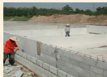
Construction of a digester at Phanus Amporn farm in Thailand
