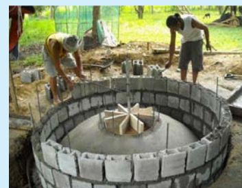
Stacked fixed dome digester construction at Nueva Vizcaya, Philippines
