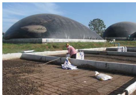
Anaerobic Digester with Solids Dry Pit in the Foreground (Thailand)
