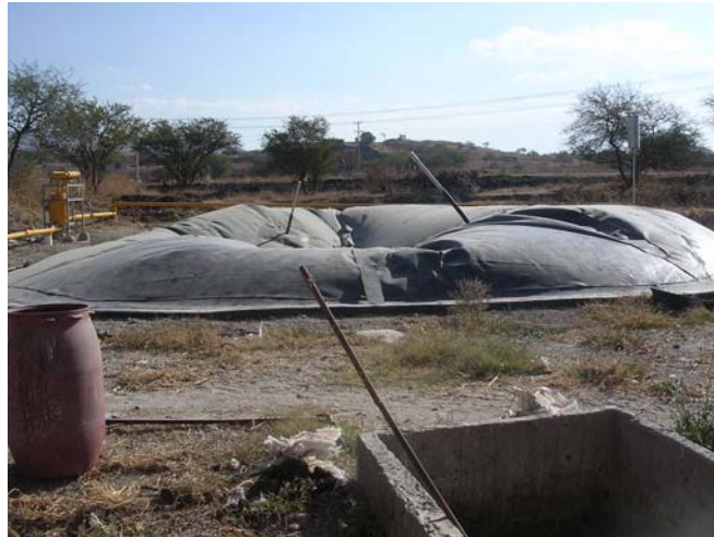
Illustration 2. Collecting Tank and Anaerobic Digester. Farm Paraíso IV. Abasolo, Guanajuato. Mexico
