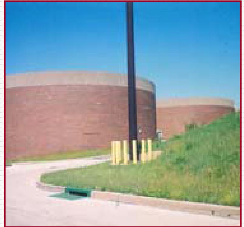
Digesters at NEWPCP are mixed by sludge circulation (sludge drawn off from the bottom of digester is mixed with feed sludge after going through a tube heat exchanger and then discharged back to digester five feet below normal liquid level)
