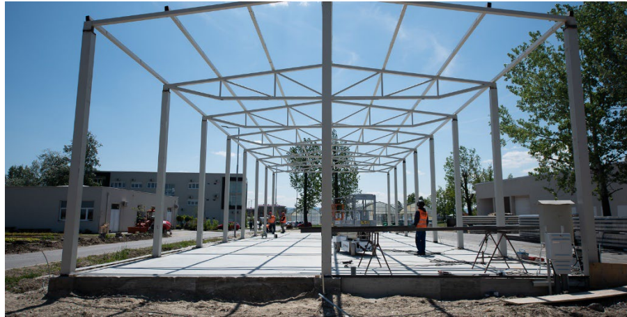
Installation of the steel structure
