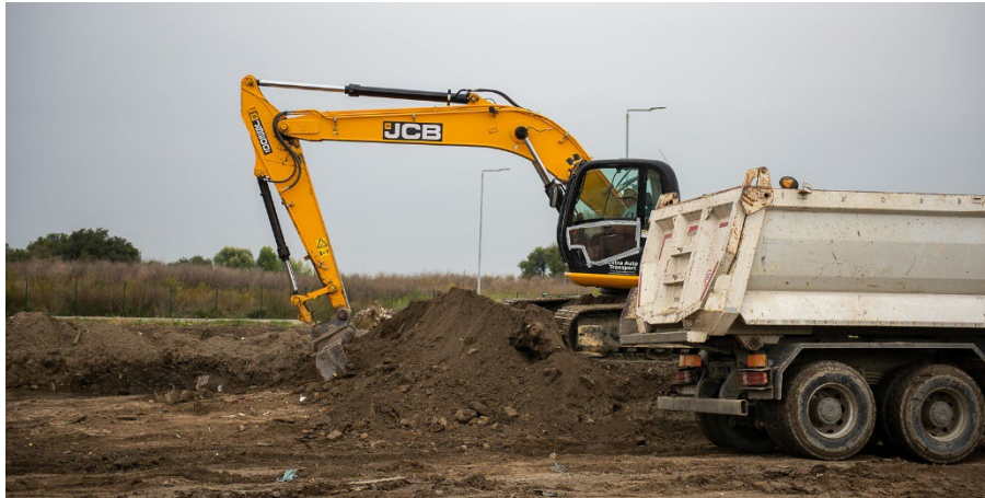
Excavation works for the plateau
