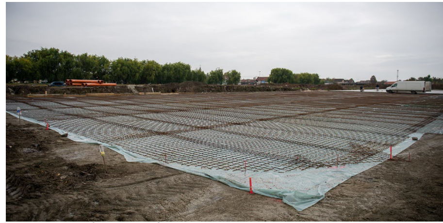
Installed reinforcement for the plateau
