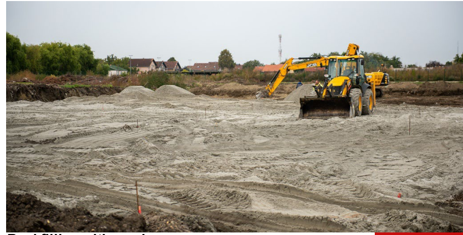
Backfilling with sand
