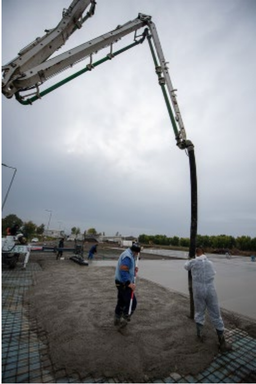
Concreting of the plateau
