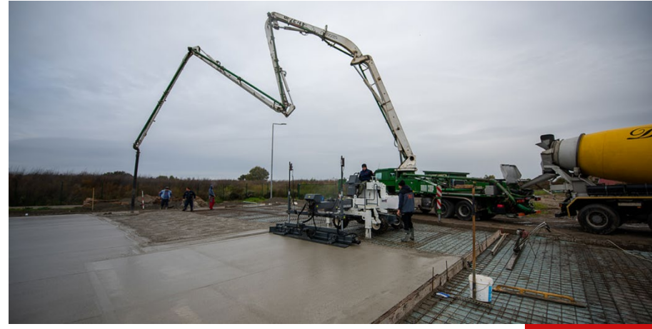
Levelling of the concrete
