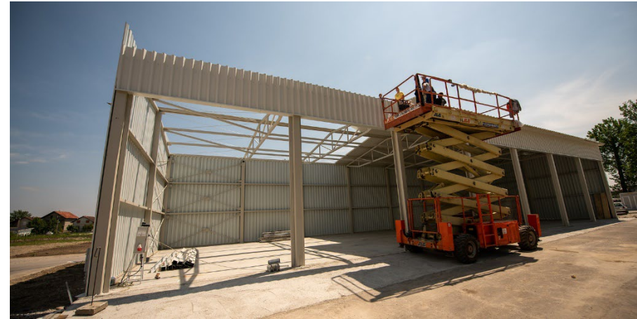
Installation of panels, roofing and roll-doors
