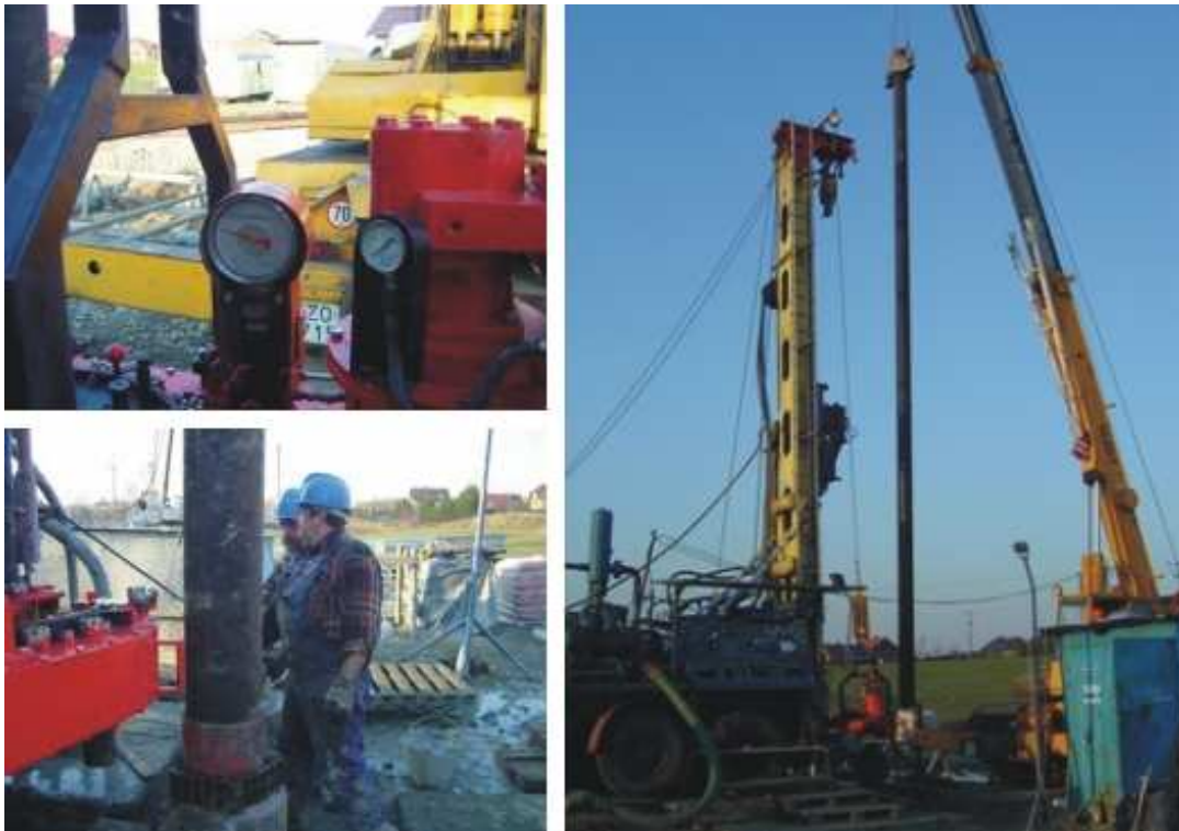
Figure 10. Installation of the Ø 244mm pipes in the borehole
