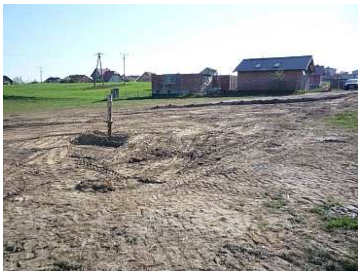
Figure 11. Site after completion of the drilling works
