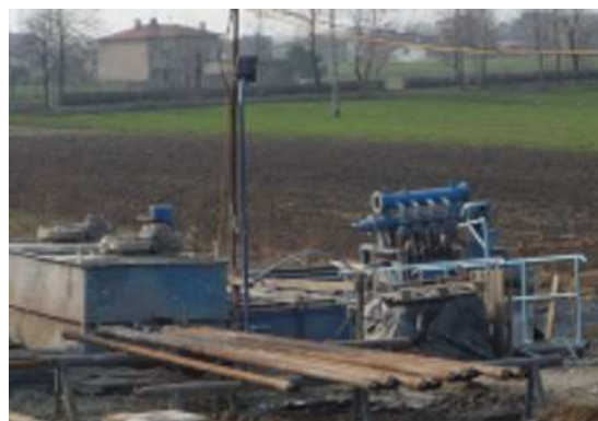
Figure 8. Drilling starting phase - general view Figure 9. Mixers and flushing pump
