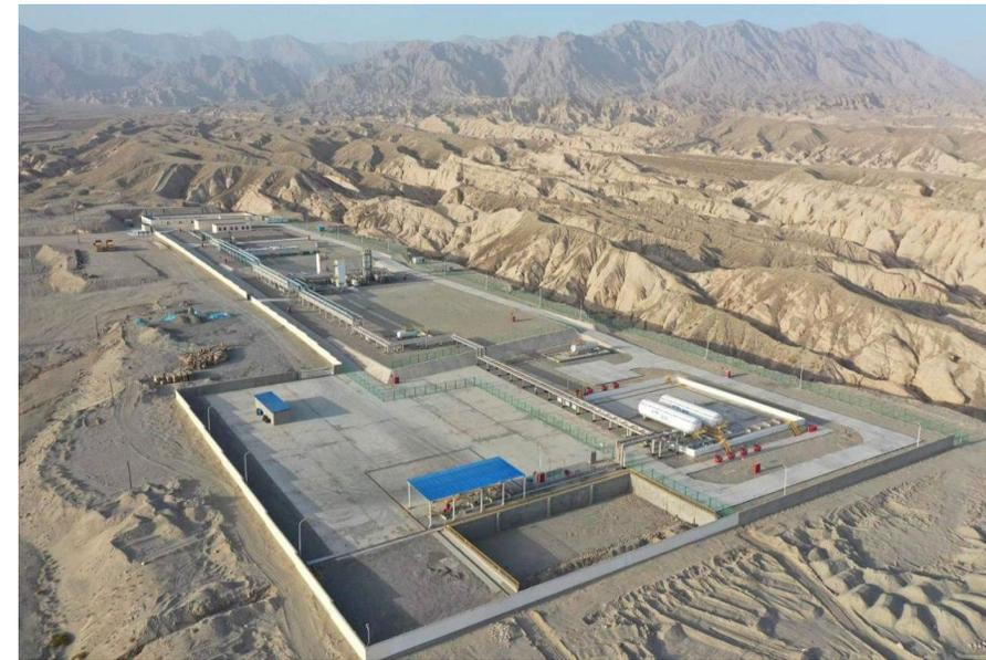
Vent gas recycling unit based on skid-mounted design + modular construction
