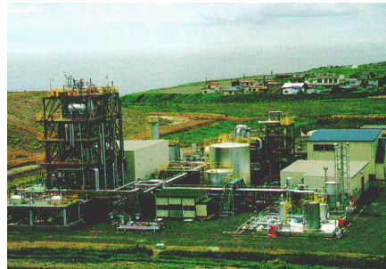
Methanol Production Plant
