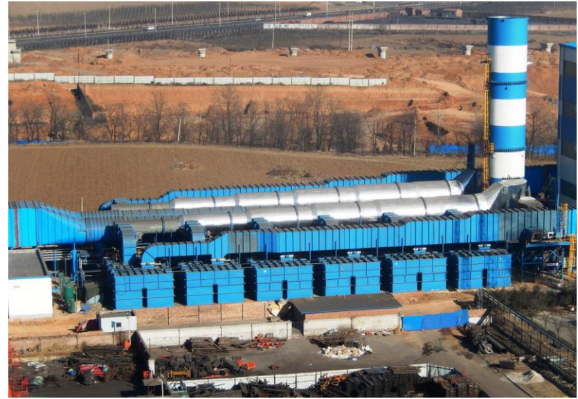
12 Regenerative Thermal Oxidizers (6 in front row)
