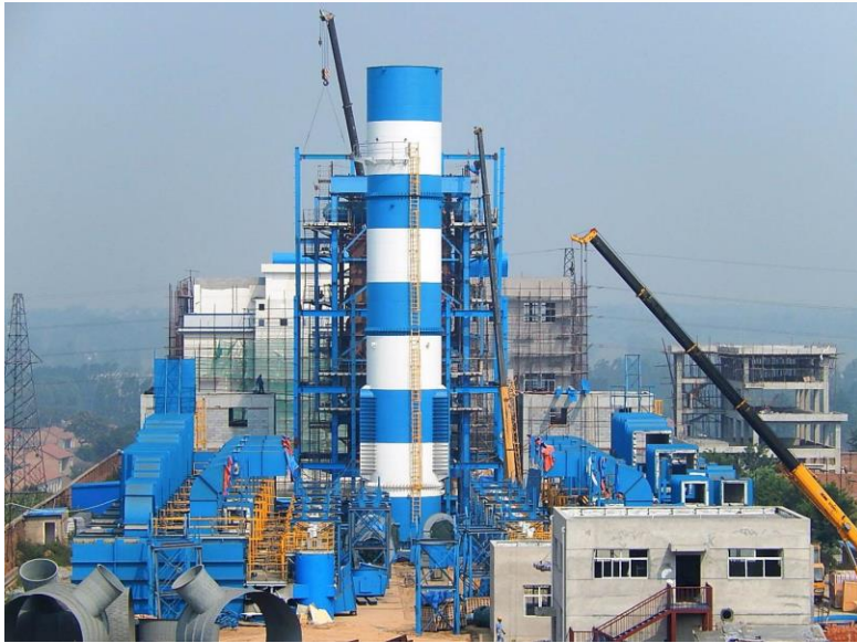
GaoHe Mine Project in Construction
