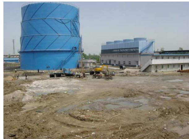
Construction Site of Demonstration Project
