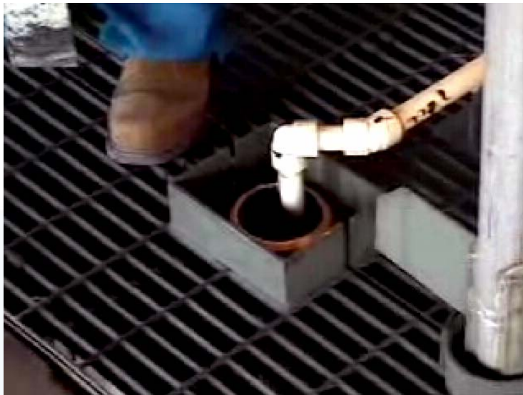
Visual image of open-ended drain
