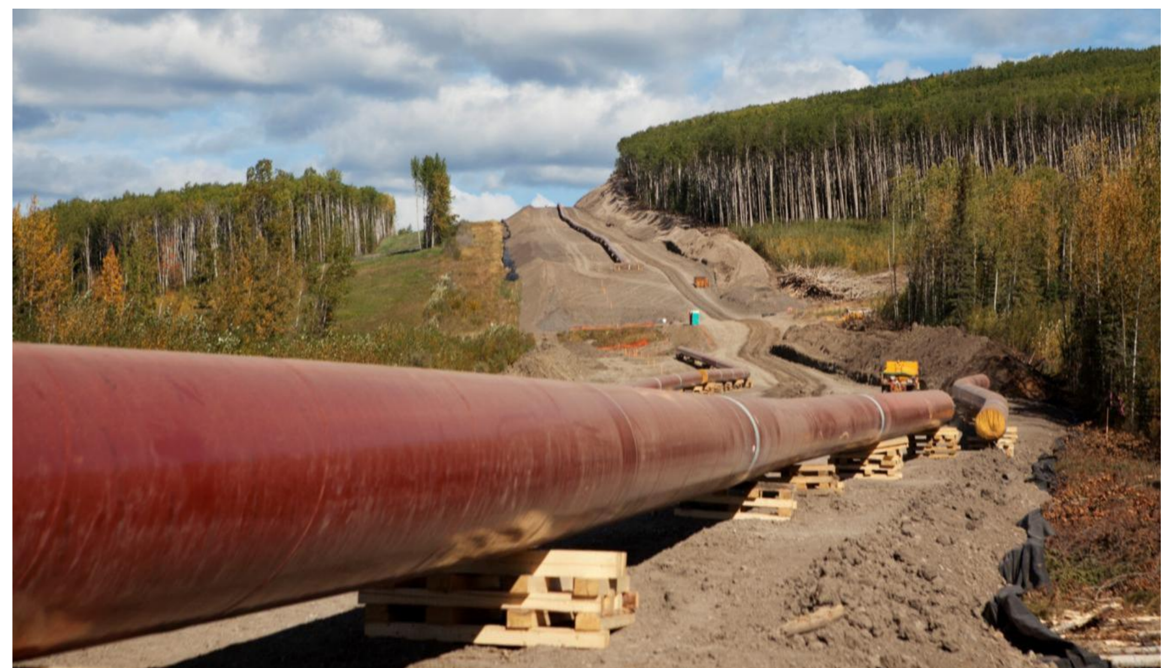
Natural gas transmission pipeline under construction in British Columbia.
