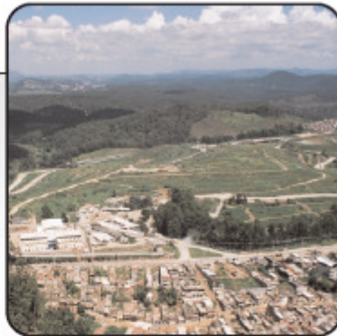
One of the world's largest single landfill-gas powered thermoelectric plants was commissioned in January 2004.
