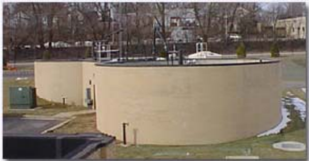
Conventional digesters (floating top)
