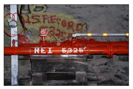
Meter Run for CMM Flow, Pressure, and Quality Measurements
