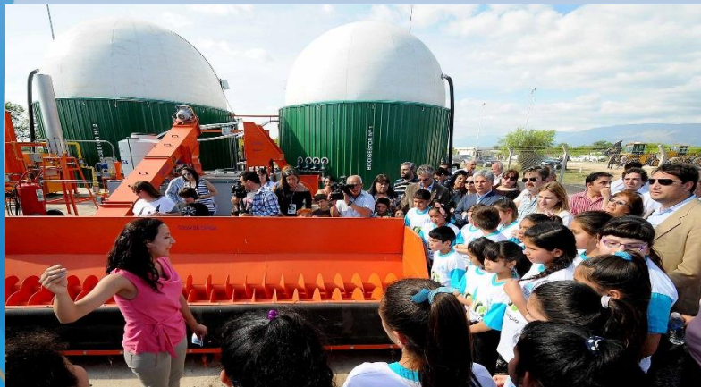
Wet residue plant in San Luis
