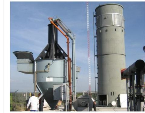
**Figure 4-5. Leachate Evaporator System at El Verde Landfill in León, Mexico**
