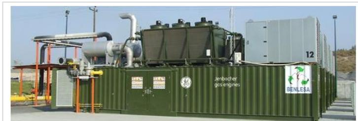
**Figure 4-6. GE Jenbacher Internal Combustion Engine at Simprodeso Landfill in Monterrey, Mexico**
