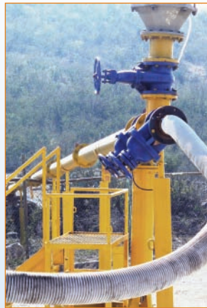
Horizontal well for extracting CMM. The extraction rate averages about 300 m 3 /s, with an average methane concentration of 80 percent.
