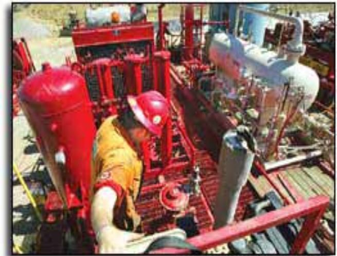
JERRY McBRIDE / Herald Portable compressors, separator and other equipment on a trailer 挂车上的便携式压缩机、分离器和其他设备
