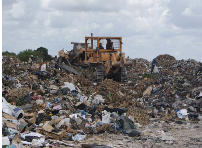
Covering waste with soil materials.
