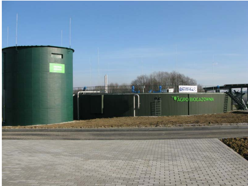
from left biogas tank, in depth fermentation reactor
