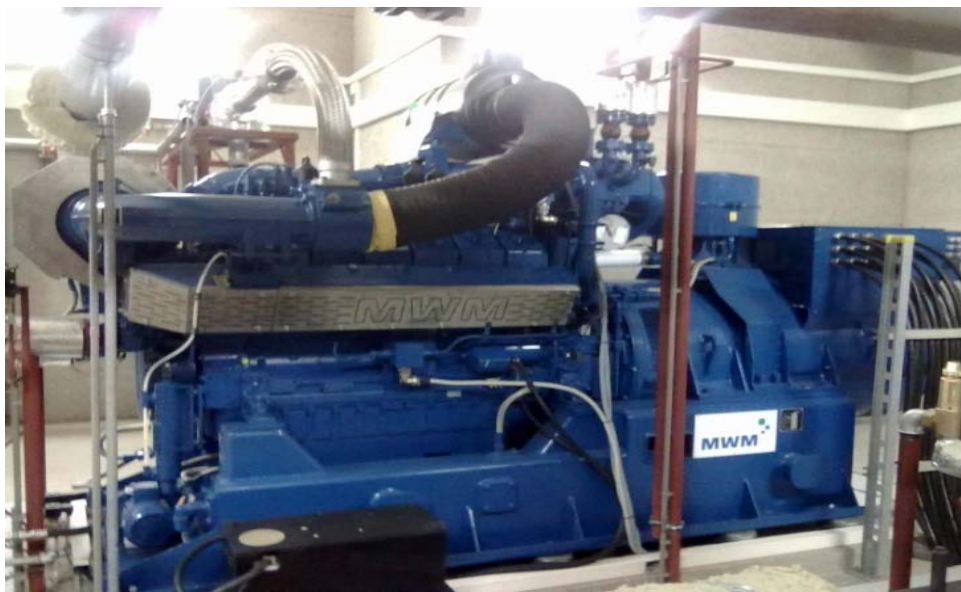
Gas engine 600 kW power
