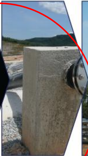
CMM Extraction and Recovery
