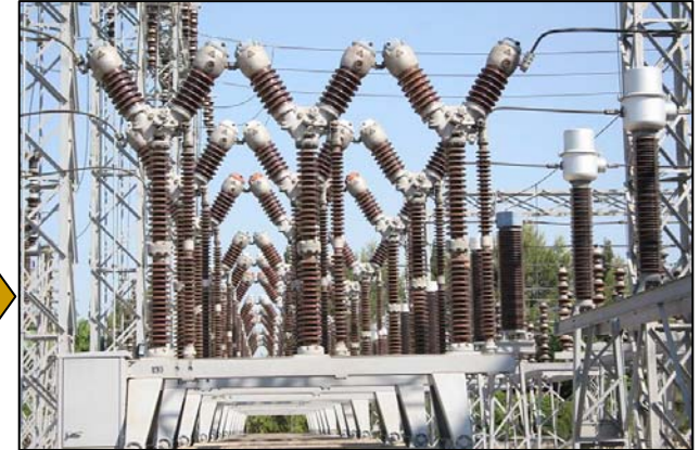
Transformers of 4,160 to 34,000 Volts
