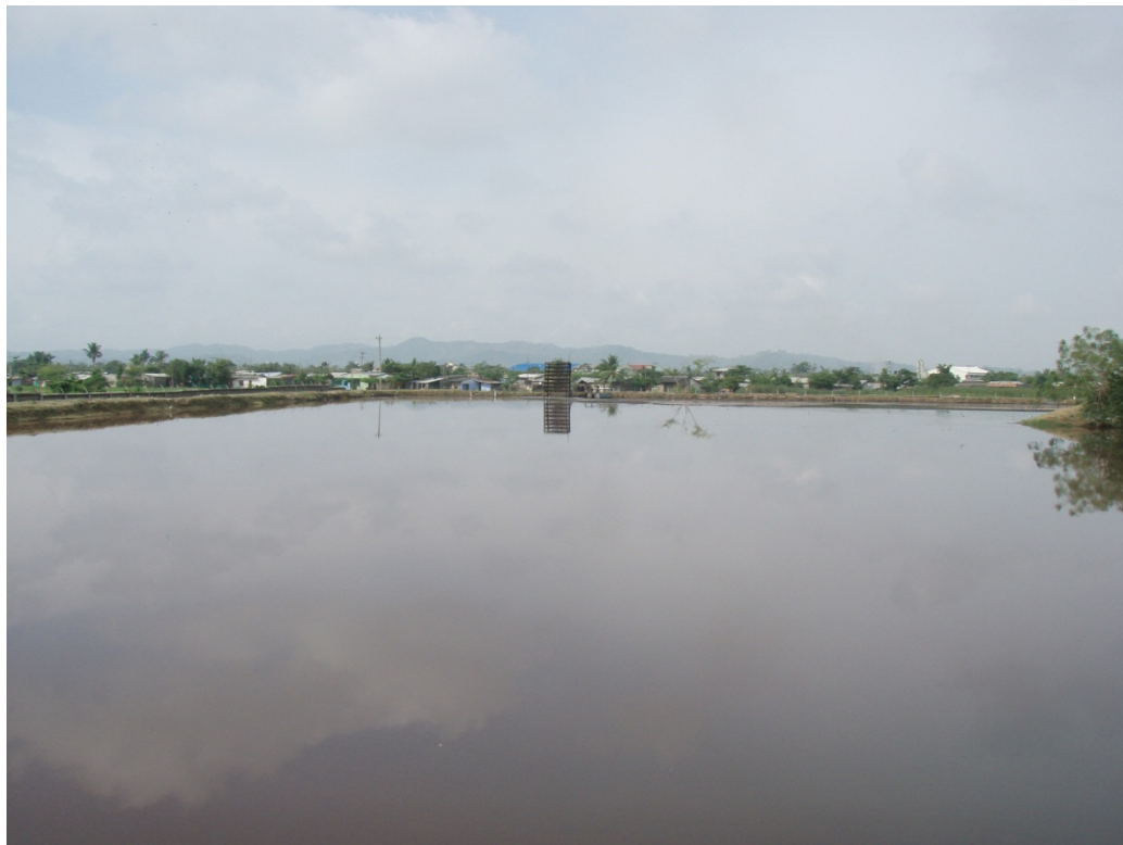
Picture 2: Second Lagoon at Frigosinú
