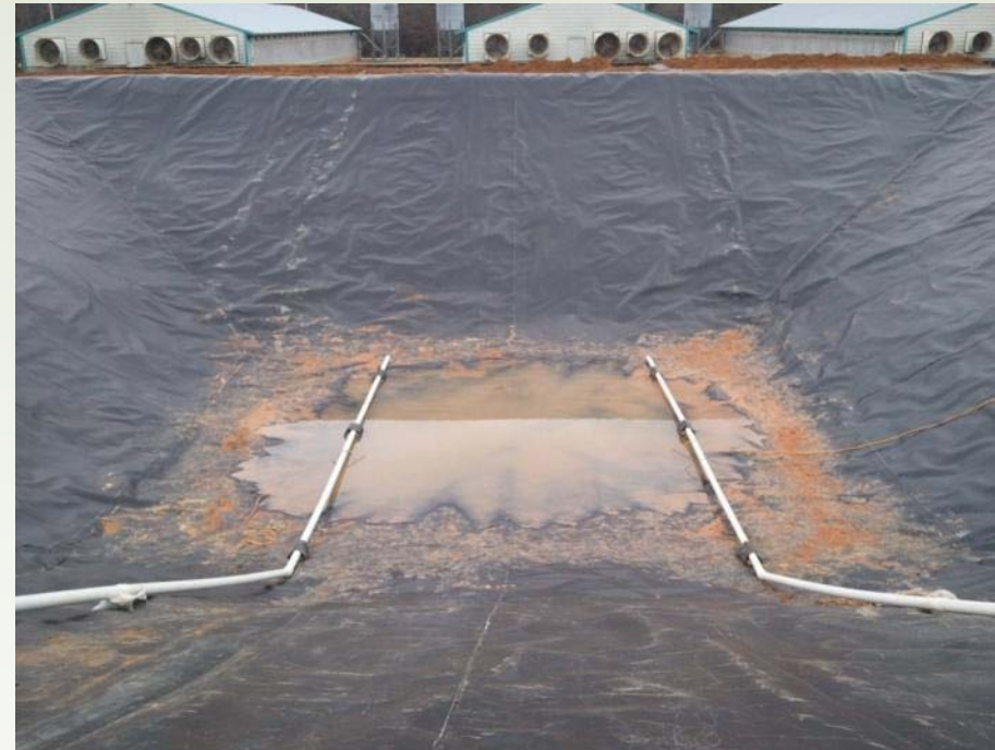
Sludge Removal System Installation
