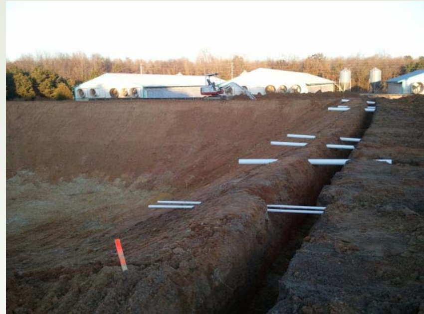
Anchor Trench and Piping
