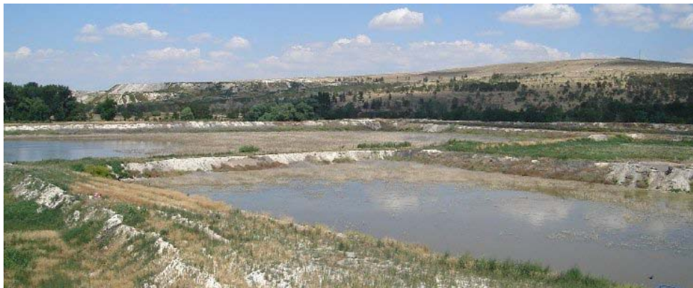
Open anaerobic lagoon at the sugar factory before a wastewater treatment plant was installed.
