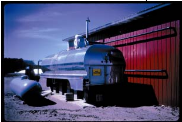
Hot Water Storage
