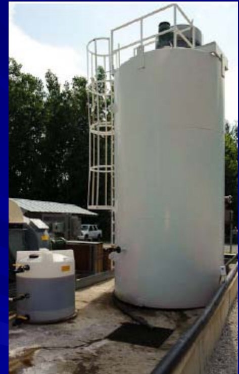
Residual From One Tank Wagon Collected In 200 Gal Poly Tank
