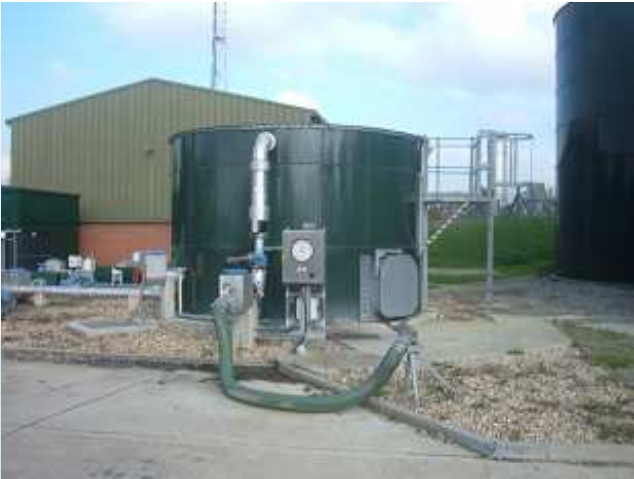
Sludge import tank
