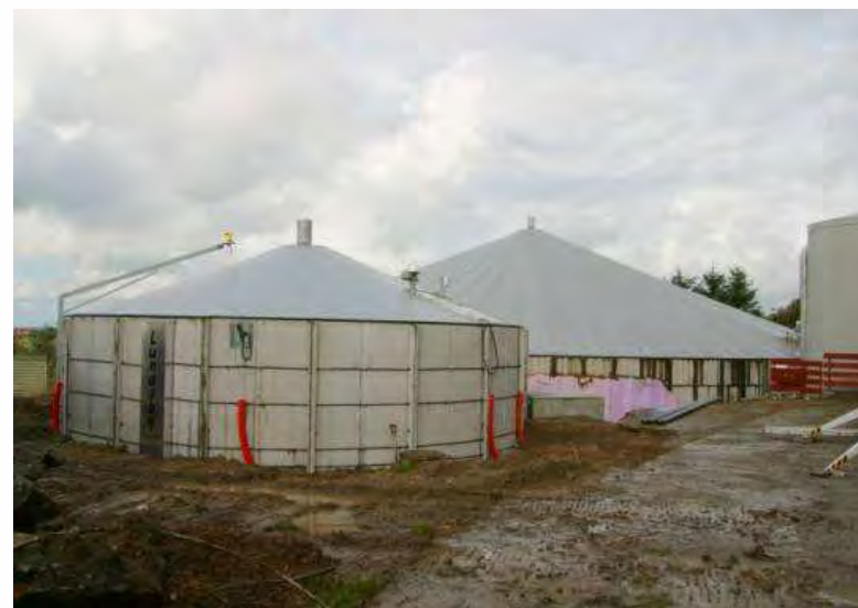
First biogas plant for manure at Jæren
