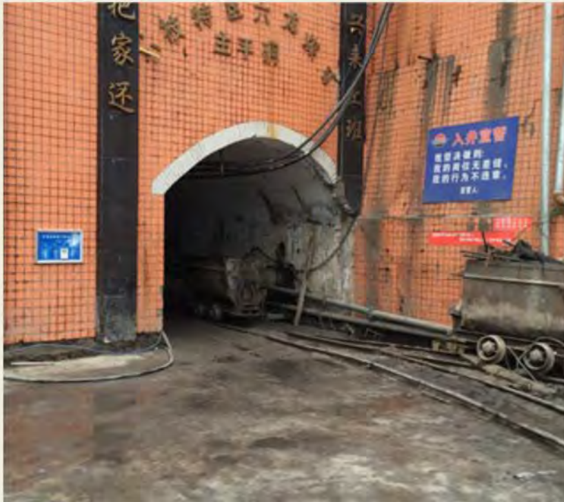
Mine Entrance, Liulong Mine, China
