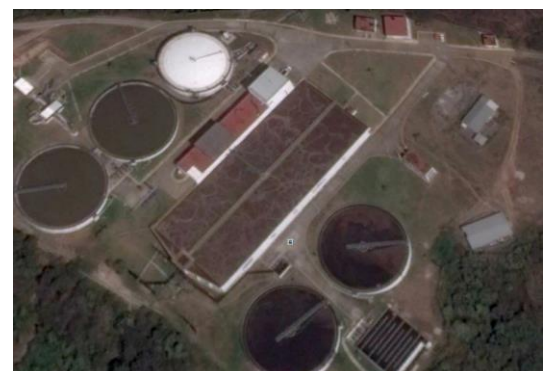
Layout of a WWTP with a CAS treatment system and primary and secondary sludge anaerobic digestion.
